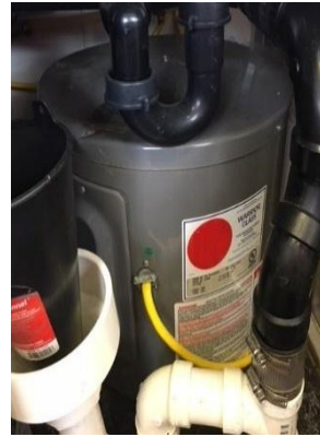
Tank water heater
