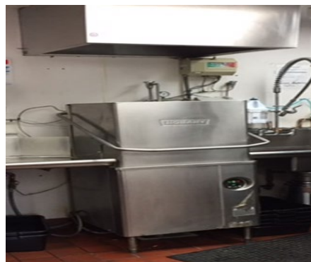
Type II hood over heat/moisture producing dishmachine
