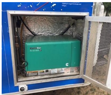
Generator installed in exterior compartment of unit
