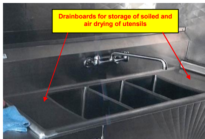
Fixed 3-compartment set up with drainboards
