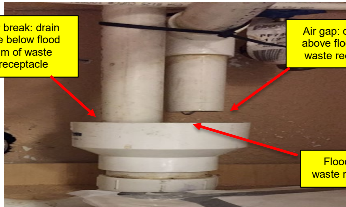
Indirect connection (air gap or air break)- permitted on equipment in which food, portable equipment or utensils are placed. Drainline off ice bins/machines must be through an air gap.
