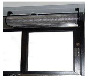
Air curtain over pass through window
